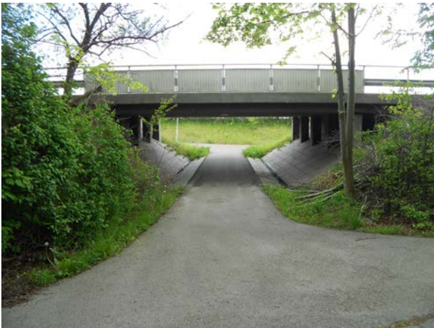
Figur 13-6. Tunnel under Fjelievägen.
